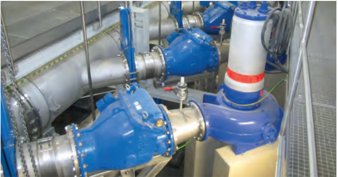
**Resilient seated disc with Stainless Steel hinge.**
