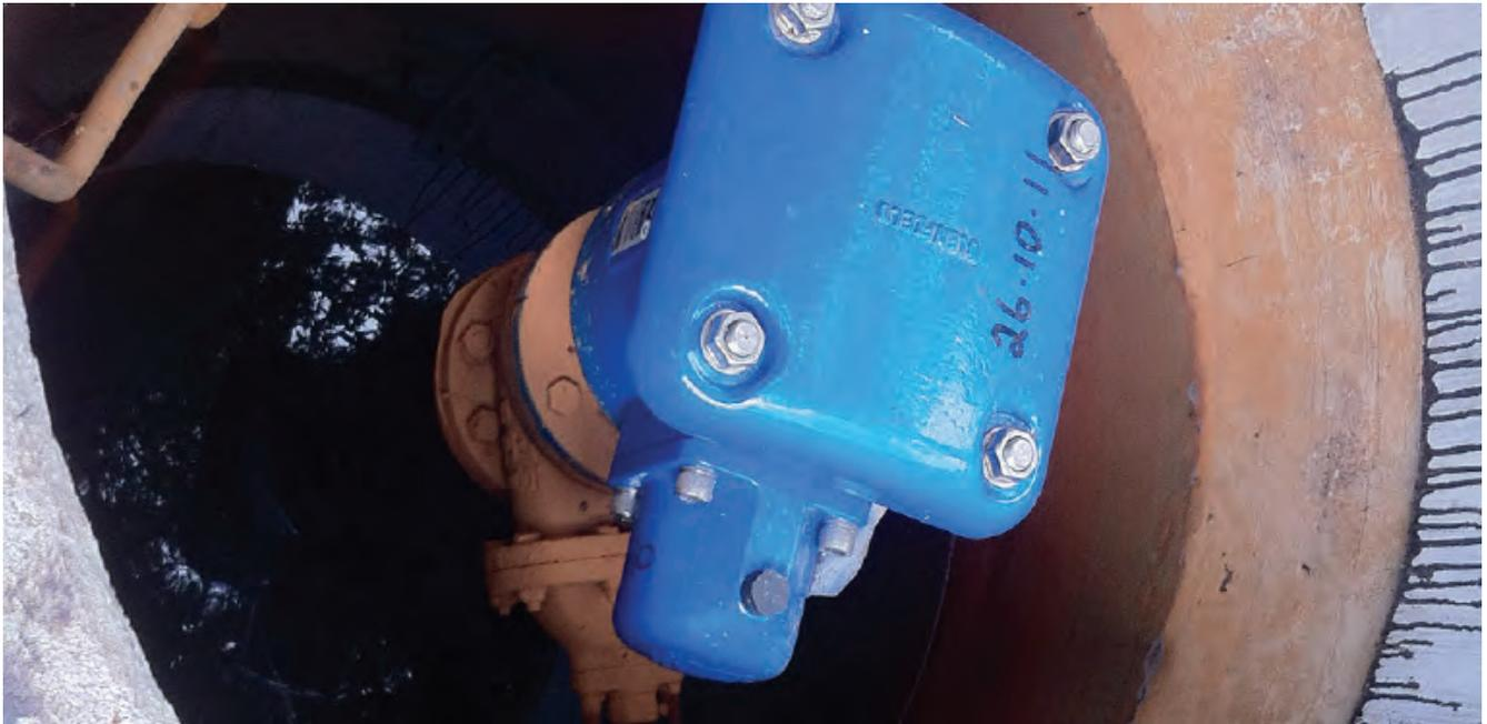
AVK's Large Orifice Series 851 Air Release Valves incorporate the exclusive Glenfield Aerokinetic Principle which prevents premature closure while air is being released from a pipeline.
