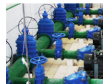
WATER PLANT WORK
