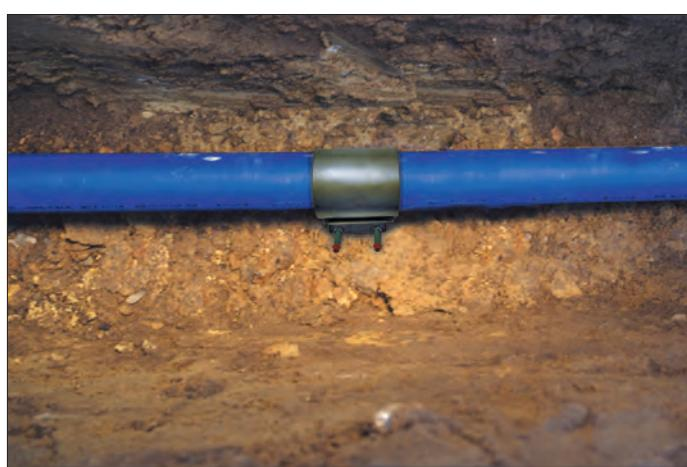
Easy and fast neutralization of the crack is essential in order to minimize disturbance for consumer. Here AVK repair clamp is mounted.
